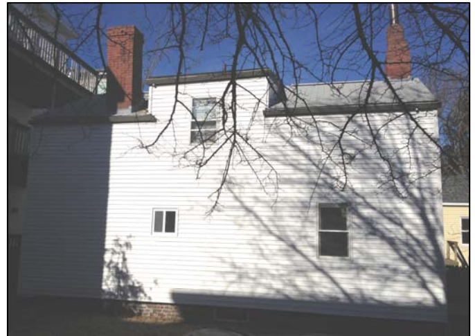
Right: Dane Street rear façade, 2014
