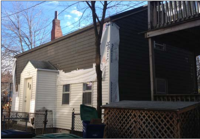
Left: Dane Street front façade 2014
