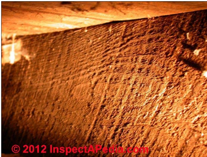
Figure 2 – Circular sawmill markings
